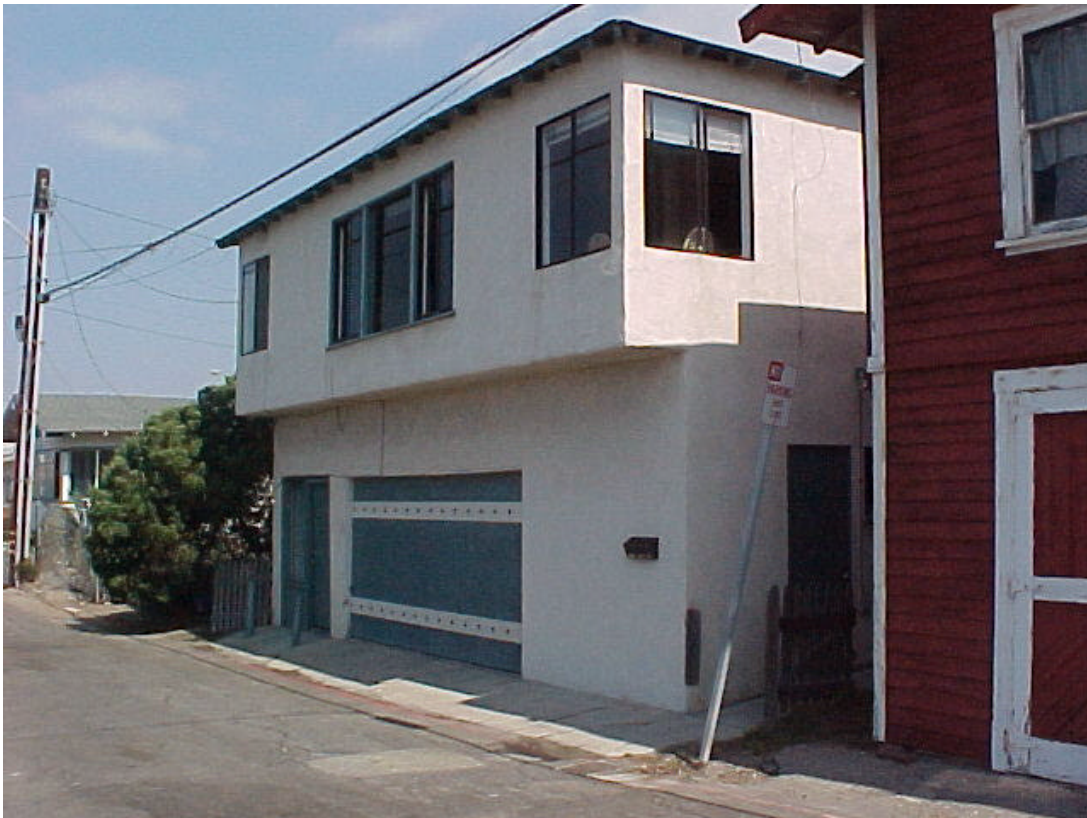
1110 Palm Drive – existing unit to be demolished and replaced
