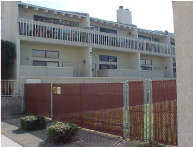
Adjacent Condos to east
