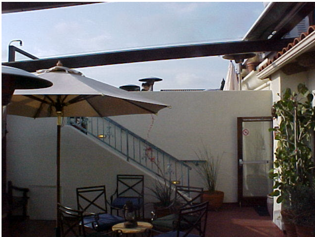
Looking up at Patio 3 from Patio 2
