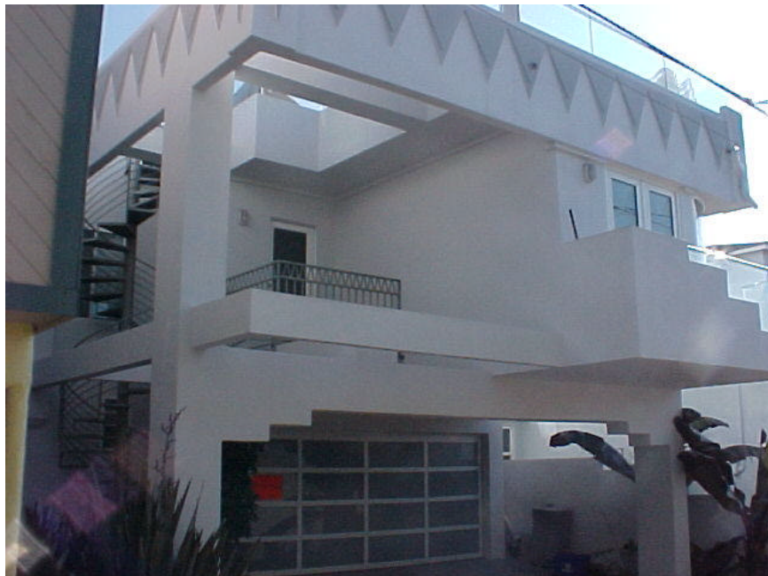
View from alley of proposed area of new construction
