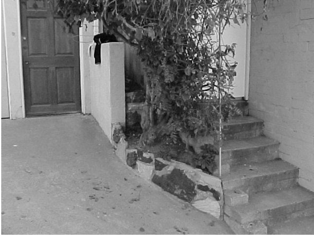
View of retaining condition at northwest property corner
