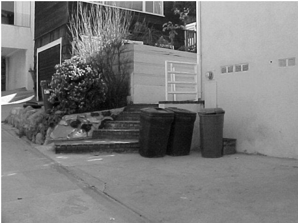
View of retaining condition at northeast property corner
