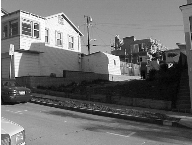
226 34 th Street – front view showing slope along eastern property line
