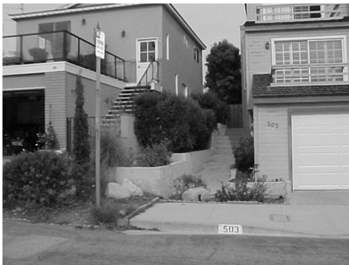
View of east property line from 24 th Street
