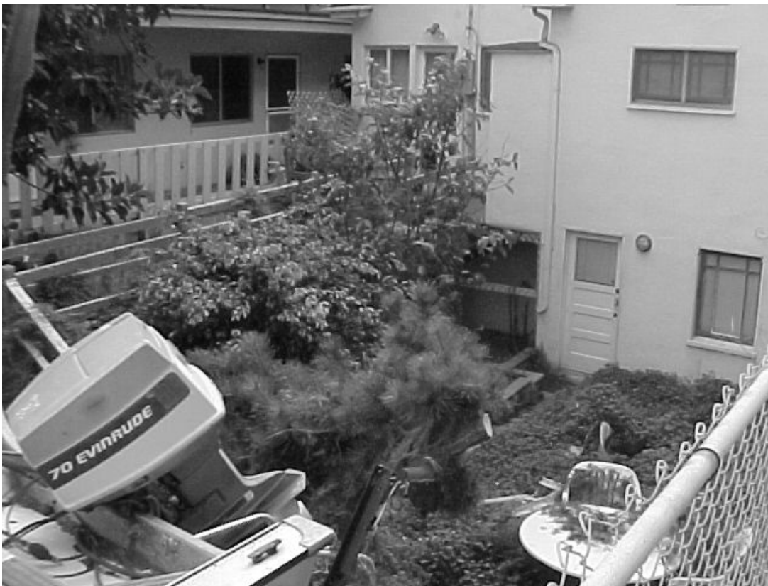
85 15 th Street – rear view showing existing basement access
