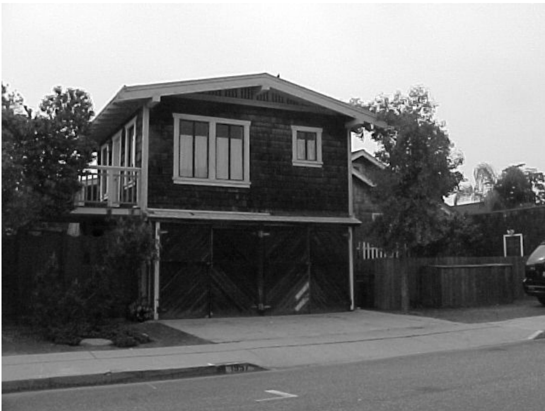
1958 Bayview Drive – view of Monterey Boulevard frontage
