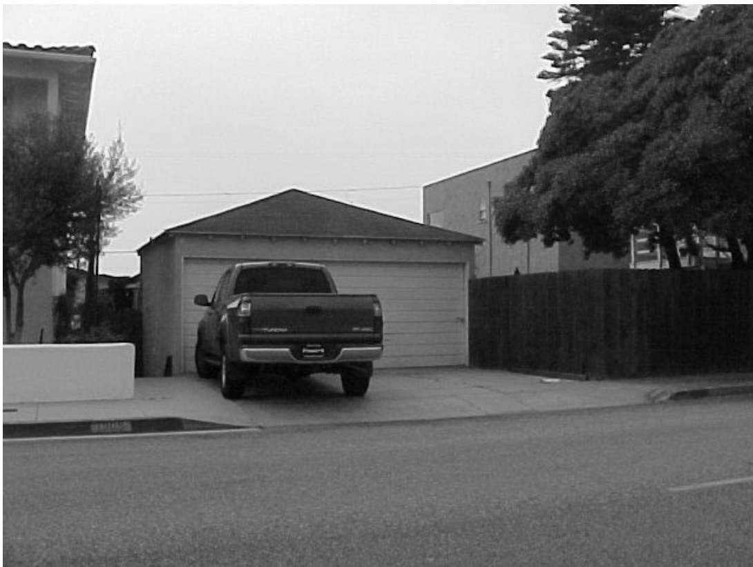
1910 Bayview Drive – view of Monterey Boulevard frontage
