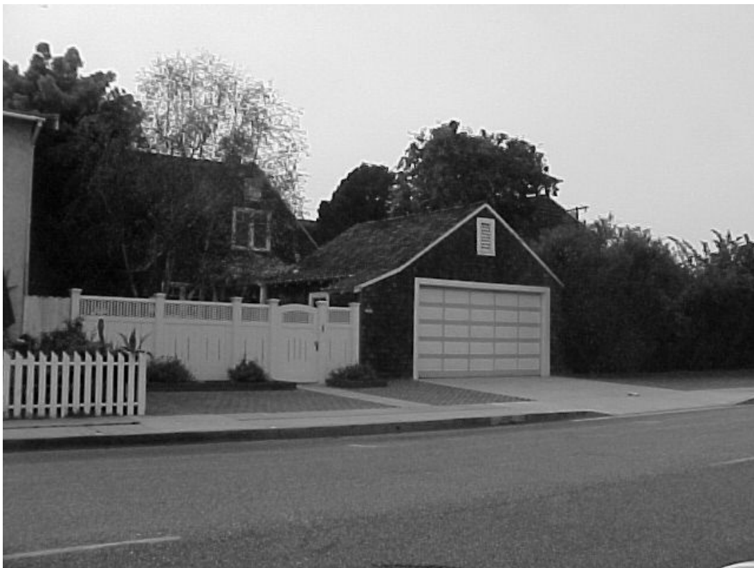
1934 Bayview Drive – view of Monterey Boulevard frontage
