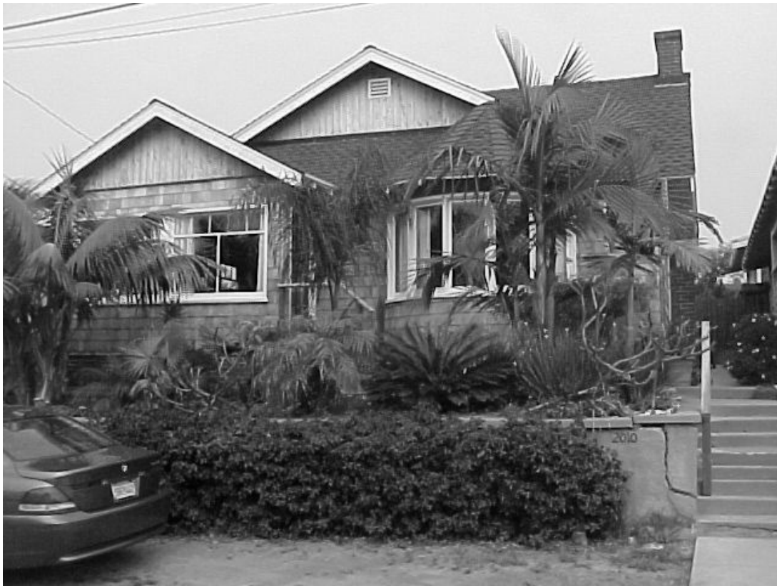
2010 Bayview Drive – view of Bayview Drive frontage
