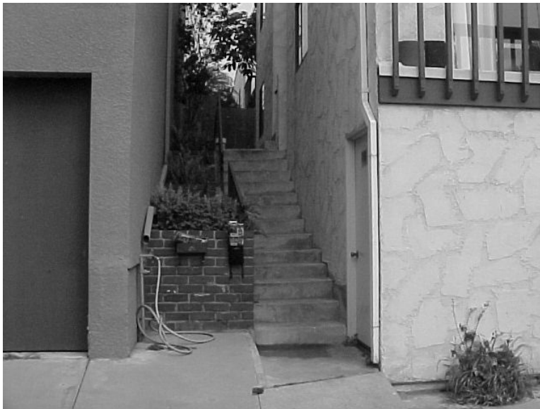
View of slope along north property line from Bayview Drive
