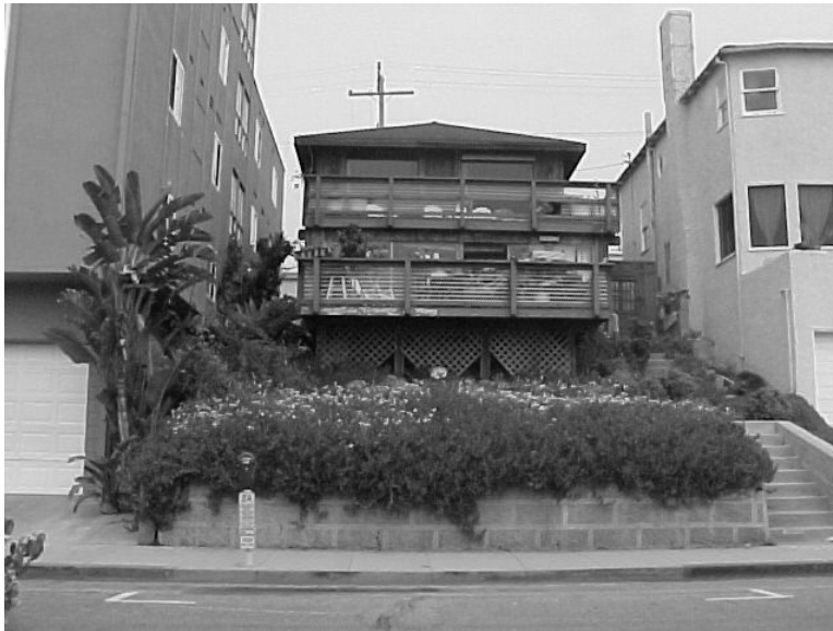
3317 Palm Drive – view from Hermosa Avenue frontage
