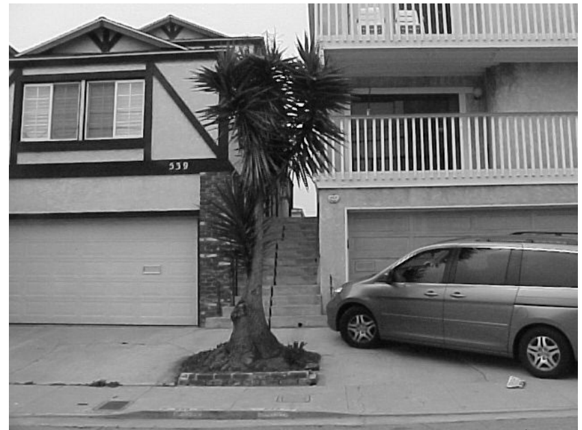
View of slope along property line between 539 and 543 2 nd Street
