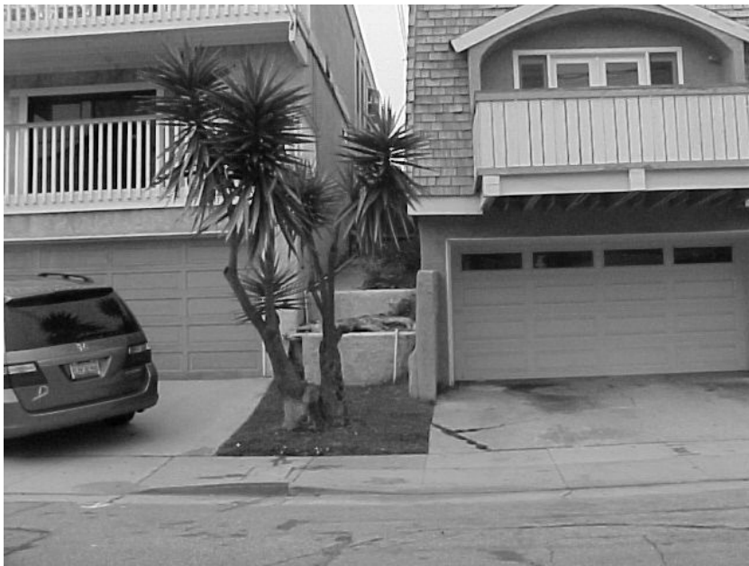
View of slope along west property line from street
