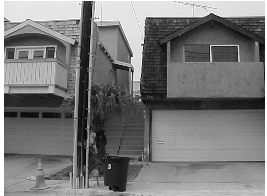
View of slope along east property line from street
