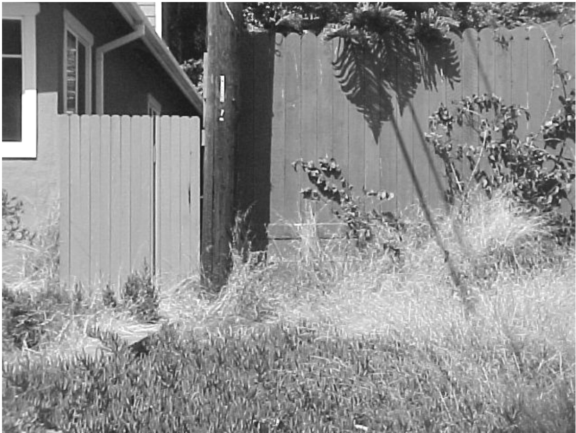
620 Gould Avenue – view of retaining wall at southwest property corner
