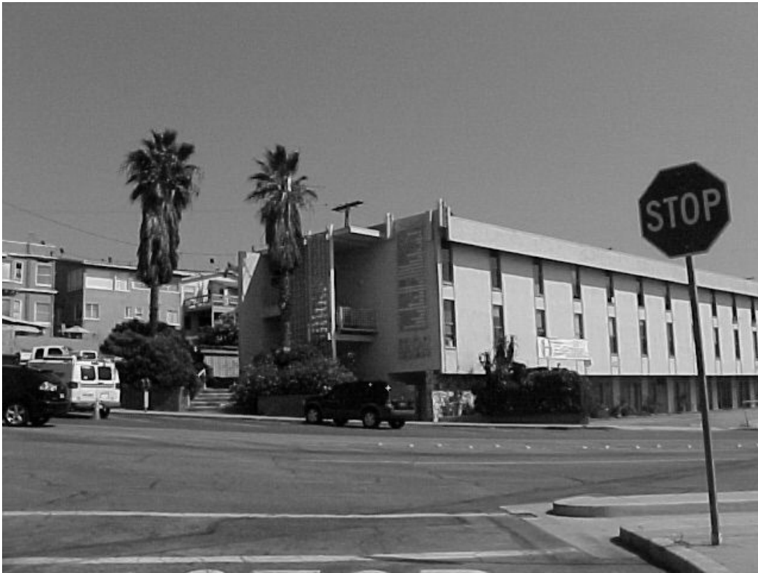
200 Pier Avenue – View of northwest corner of existing commercial building
