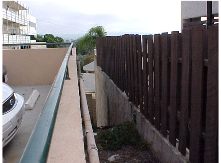
Looking South from hotel parking structure side
