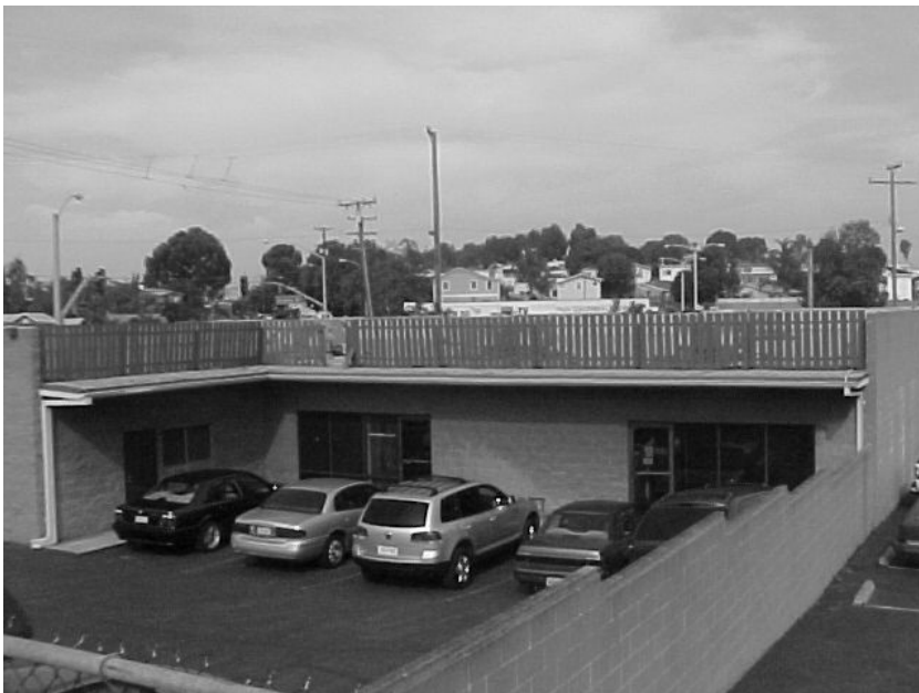
1102 Aviation Blvd. – view of Aviation Blvd. frontage from southeast (rear) property corner
