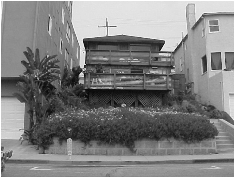
3317 Palm Drive – view from Hermosa Avenue frontage
