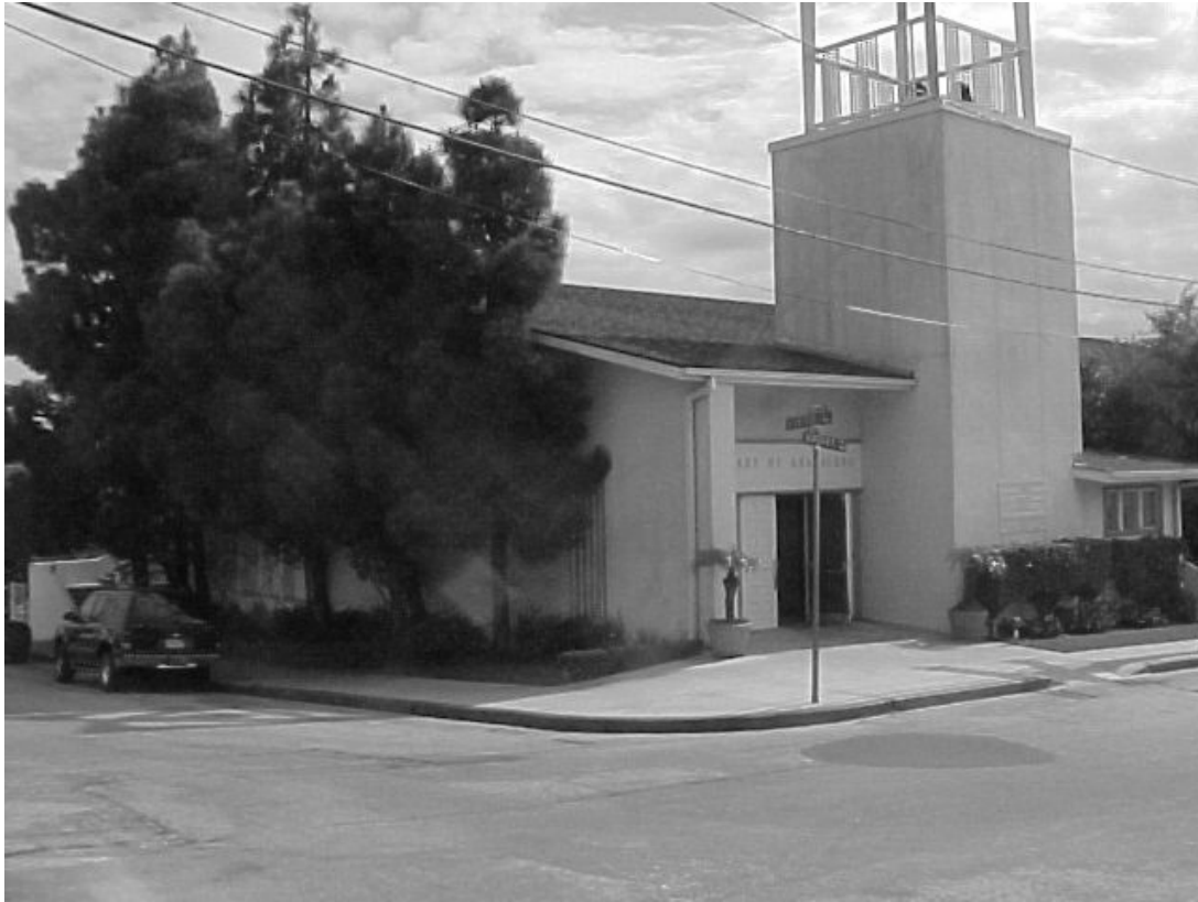
320 & 440 Massey Avenue – View of church from corner of 5 th and Massey Avenue
