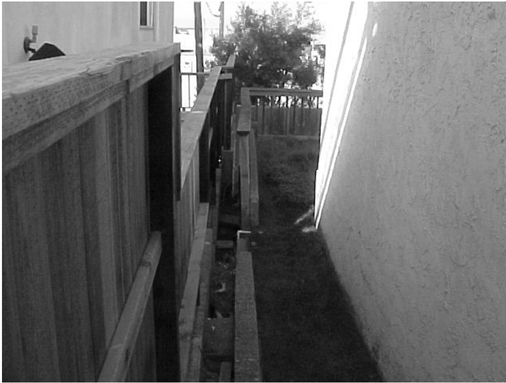
535 Gravely Court – View along south property line looking west
