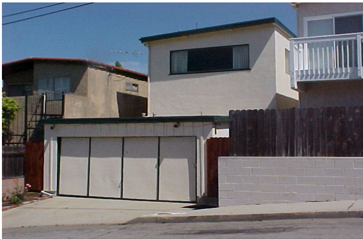
Rear view of 1222 2 nd Street, 152 square ft of addition is proposed above the existing garage.
