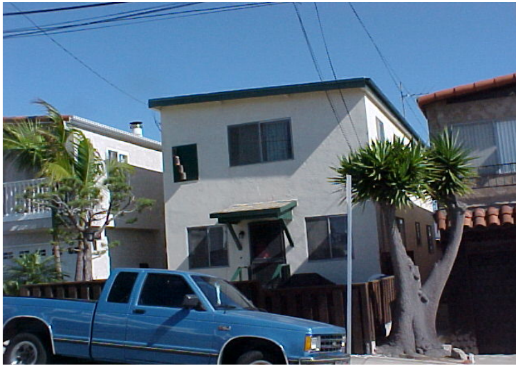
Front view of 1222 6 th Street.
