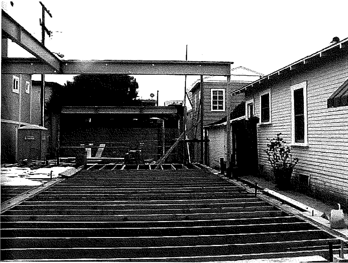
June 19, 2006 – All old framing has been removed from foundation at 311 31 st St. – red tag is posted.
