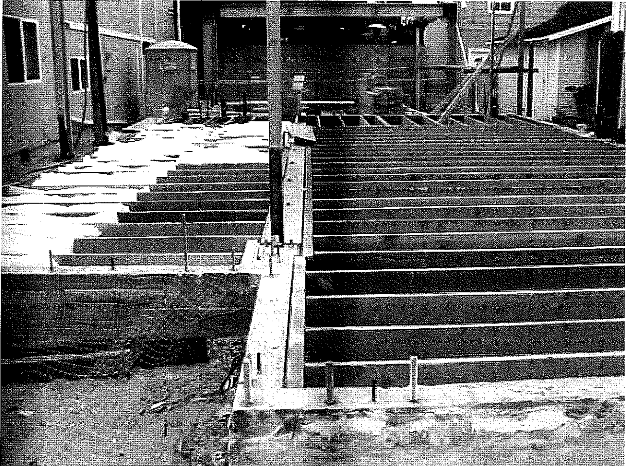
June 19, 2006 – 311 31 st St. – Some insulation has been added to floor joists. Plans show joists mounted to a sill plate, they are installed with hangers. Below, none of the original wood framework remains.
