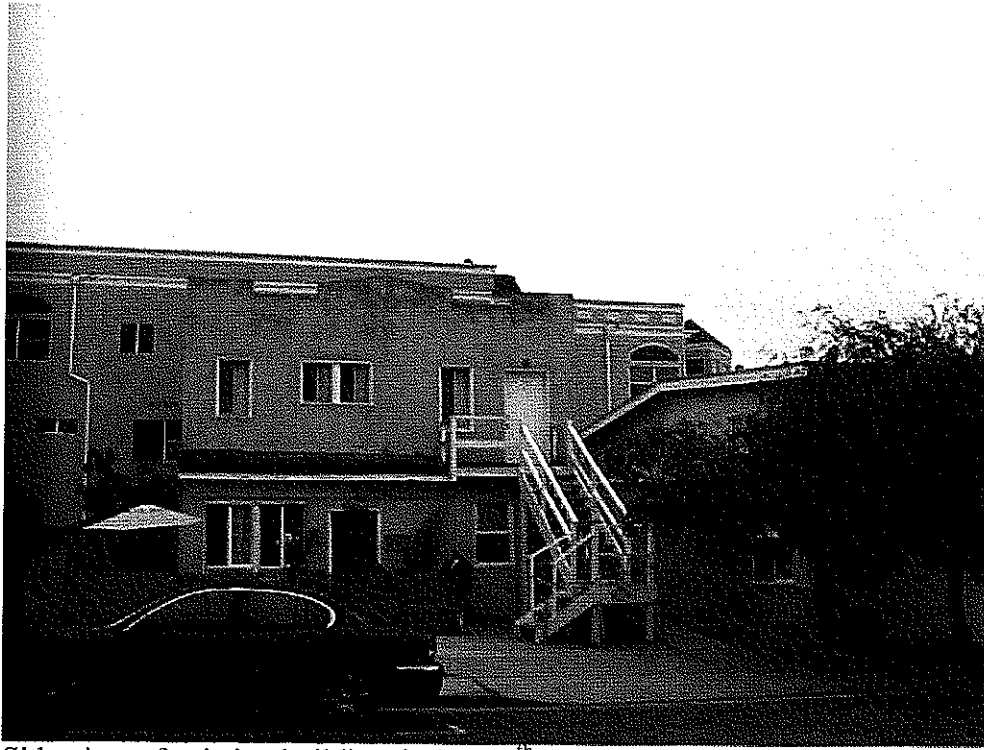
Side view of existing building facing 11 th Street.
