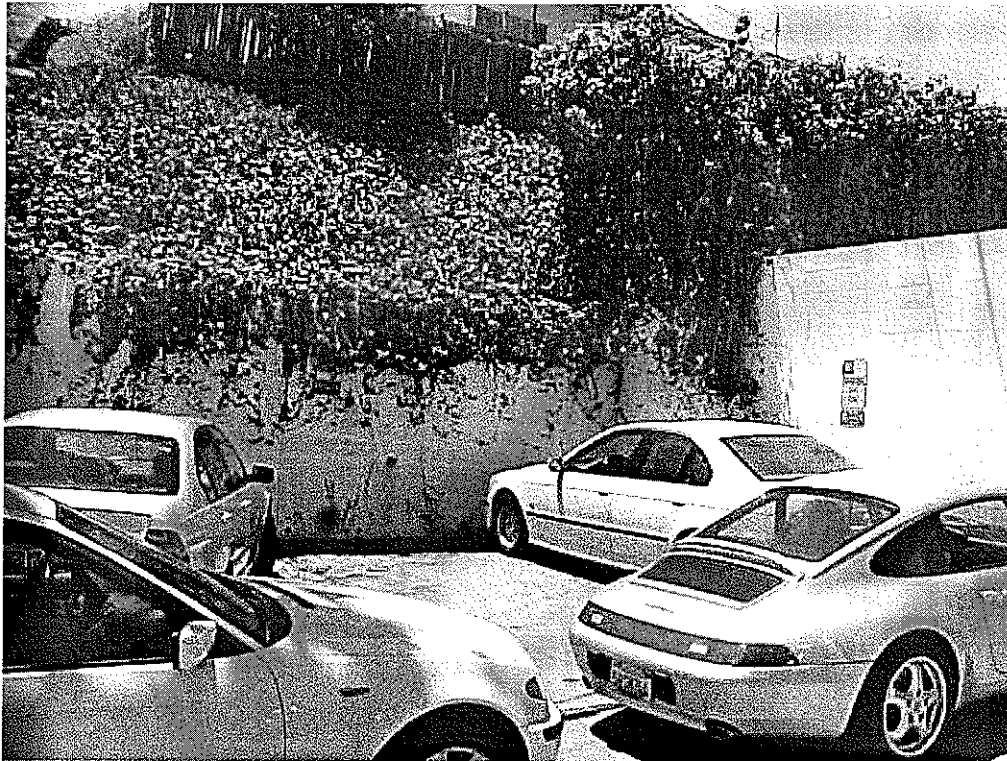
1. SOUTHERN PORTION OF LOT AT 2901 PCH THAT IS SUBJECT TO LLA
