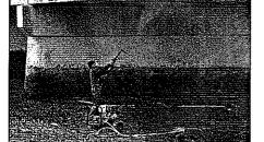
Once the patch work and repairs to the spalled areas was complete, the scope of work called for Surtreat's certified applicators to clean the concrete surfaces to remove surface chlorides, grime and debris. This was done with a high pressured power washer. Once cleaned the application of Surtreat formulations began The work was completed in five days.
