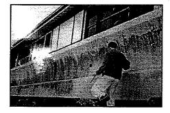
The final application consisted of a formulation that was designed to provide the greatest level of protection near the surface. This was important in providing resistance to acids and chemicals in the surrounding environment. Once again, this application was completed using spray units and pressure fed rollers.
