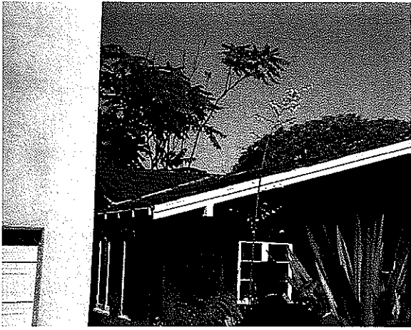
June 21, 2005 – 1811 Manhattan – Roof materials are damaged and missing, gaps in siding.
