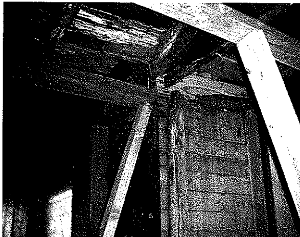
Interior photos show rotted framing members propped into place, collapsed ceiling.
