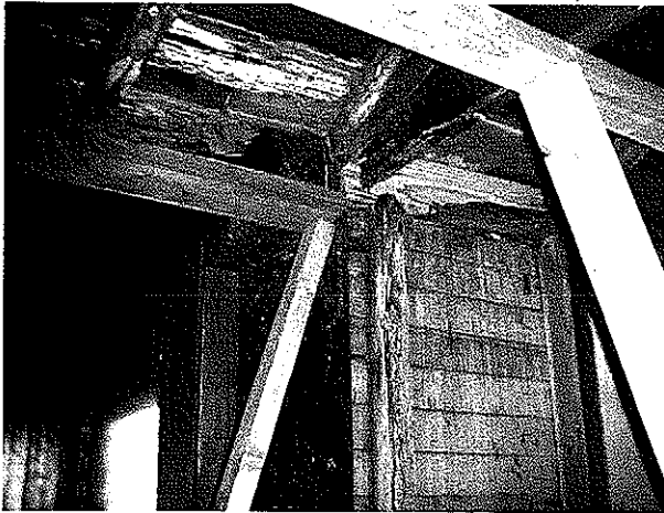
Gaps in roof, water damage and mold under windows.
