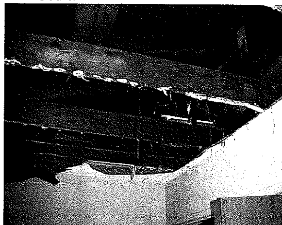
Interior photos show rotted framing members propped into place, collapsed ceiling.
