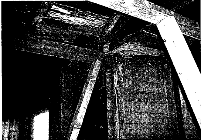
Gaps in roof, water damage and mold under windows – all photos from front unit.
