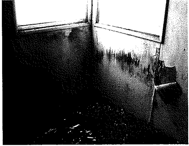
Gaps in roof, water damage and mold under windows – all photos from front unit.
