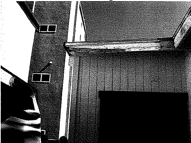
Below, rot and termite damage in eaves and rafter tails.
